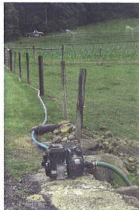
IRRIGATION AND SOLUTION TRANSFER
