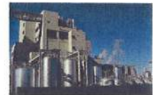
INDUSTRIAL AND WASTE TREATMENT
